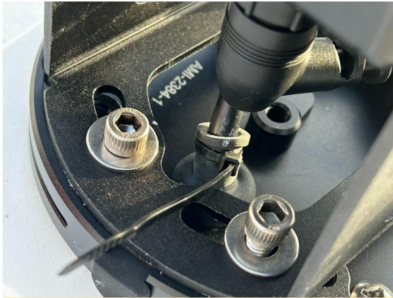
Figure 29: Cable Zip Tie Installation
